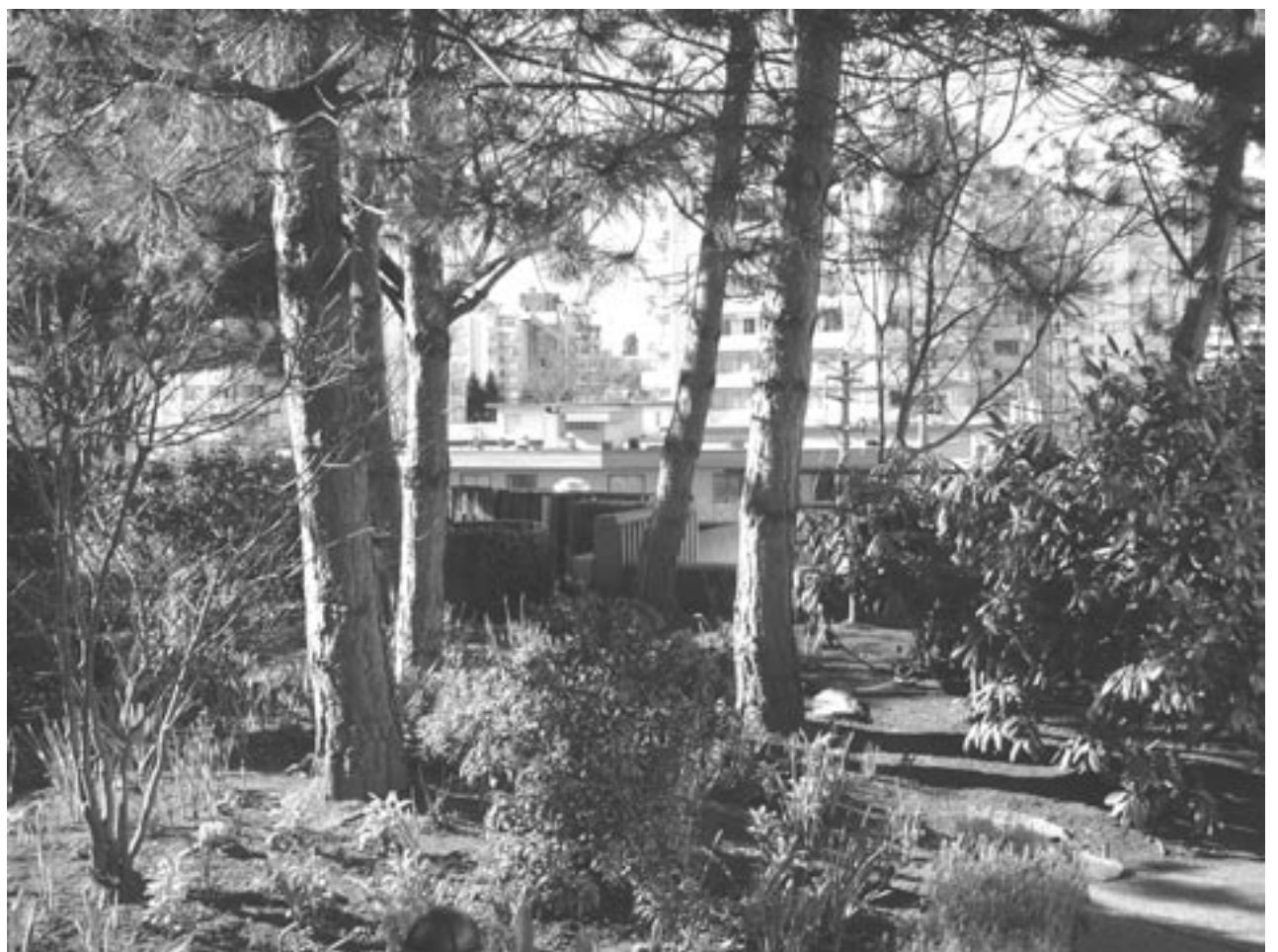
An intensive green roof atop the Coast Plaza Hotel in Vancouver, British Columbia
