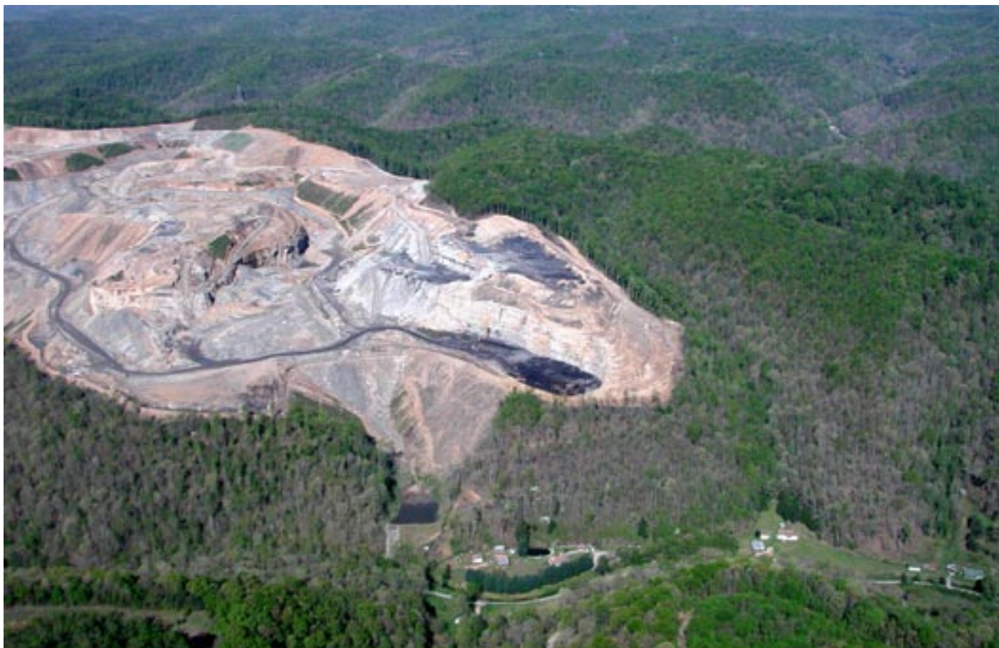
Mountaintop removal coal mine in southern WV encroaching on a small community.
